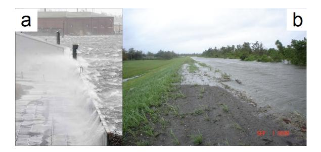
Figure 5.2. Photographs during Gustav of (a) waves overtopping the IHNC walls near the Ninth Ward, and (b) surge overtopping the earthen levee near Braithwaite (right), courtesy of Nancy Powell, USACE.
