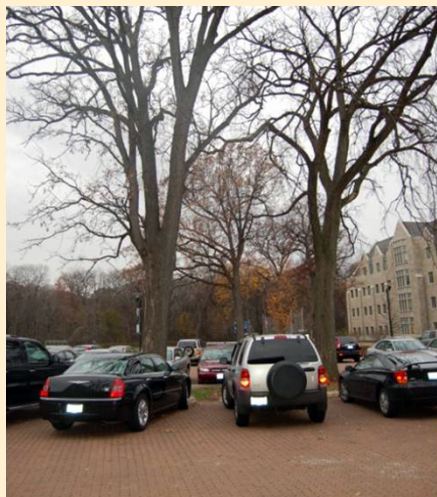
Figure 2. Leaf and tree detritus collects in pathways intended for water in PICP located underneath a tree line outside Chicago, IL.
