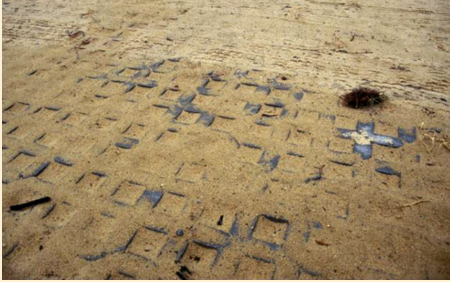
Figure 6. Mechanical sweeper bristle penetration of larger gaps associated with CGP filled with sand (left) is possible, but pavement types with small gaps (such as PICP) is not (right, courtesy of Elgin Street Sweepers).
