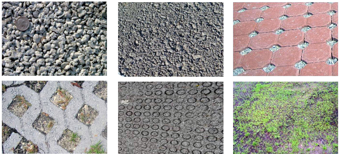
Figure 1. Types of permeable pavement. Top L-R: Permeable concrete (PC), permeable asphalt (PA), permeable interlocking concrete pavers (PICP). Bottom L-R: concrete grid pavers (CGP), plastic reinforcing grids (PG) filled with gravel, and PG with grass.
