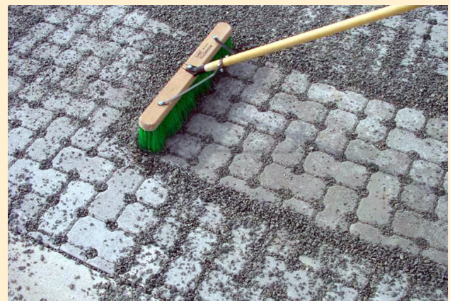
Figure 8. PICP gaps must be filled with aggregate to prevent a tripping hazard (top). Gravel replacement is simple and done with a push broom (bottom).
