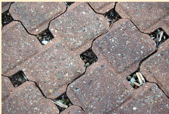
Figure 2. Leaf and tree detritus collects in pathways intended for water in PICP located underneath a tree line outside Chicago, IL.
