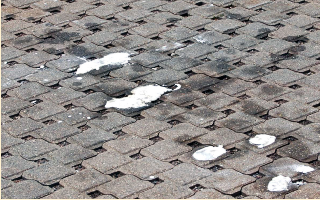
Figure 9. A stain remover applied to PICP (left) and subsequent pressure washing (right). Ideally, the stain remover is allowed to set overnight.
