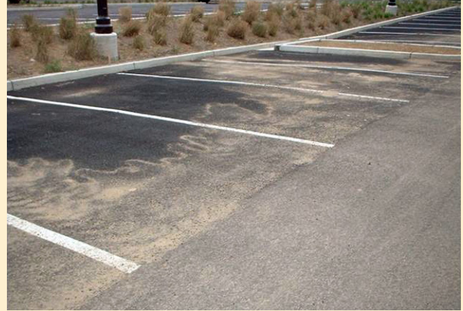
Figure 3. Residential construction increases the likelihood of sediment accumulation in permeable pavements (left). A pervious asphalt pavement near Philadelphia, PA, is clogged due to runoff from an adjoining area that was not stabilized (right).
