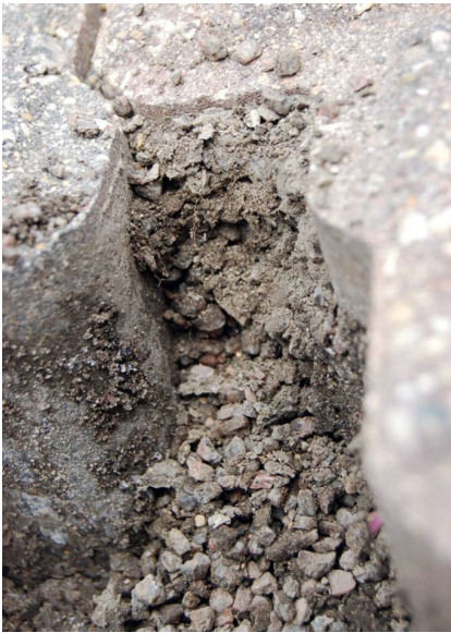
Figure 7. The clogged zone of PICP is evident toward the top portion of the interlocking paver. The depth of clogging at this location outside Chicago, IL, after 6 years of neglect was 1.5 inches (40mm).
