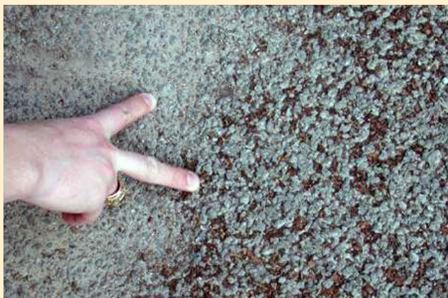
Figure 4. Visual inspection of a pervious concrete lot in Georgia shows accumulation of both sediment and leaf debris (left). The fact that the lot is clogged is confirmed by emptying approximately 1 gallon of water on the lot, which subsequently runs off rather than infiltrating (right).
