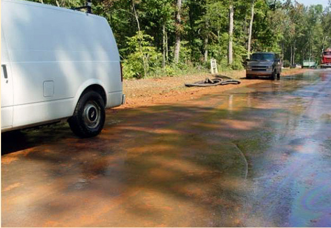
Figure 3. Residential construction increases the likelihood of sediment accumulation in permeable pavements (left). A pervious asphalt pavement near Philadelphia, PA, is clogged due to runoff from an adjoining area that was not stabilized (right).
