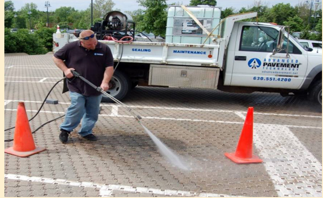
Figure 9. A stain remover applied to PICP (left) and subsequent pressure washing (right). Ideally, the stain remover is allowed to set overnight.
